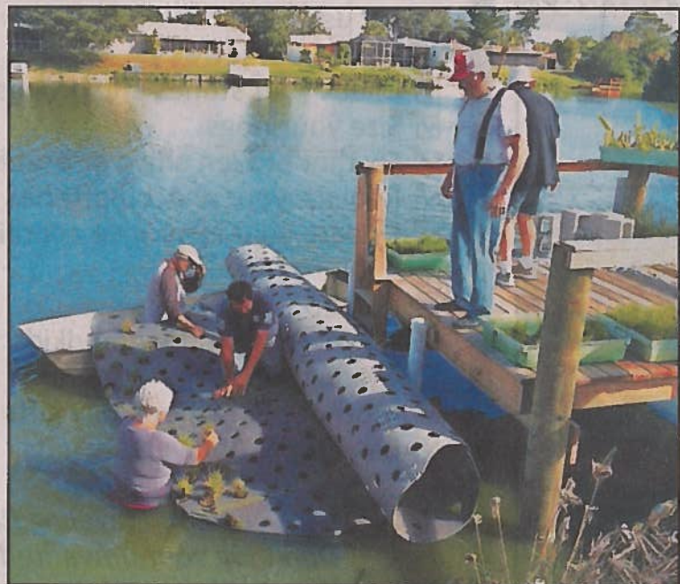
The floating island is a 256-square-foot mat, which has been plugged with plants.
