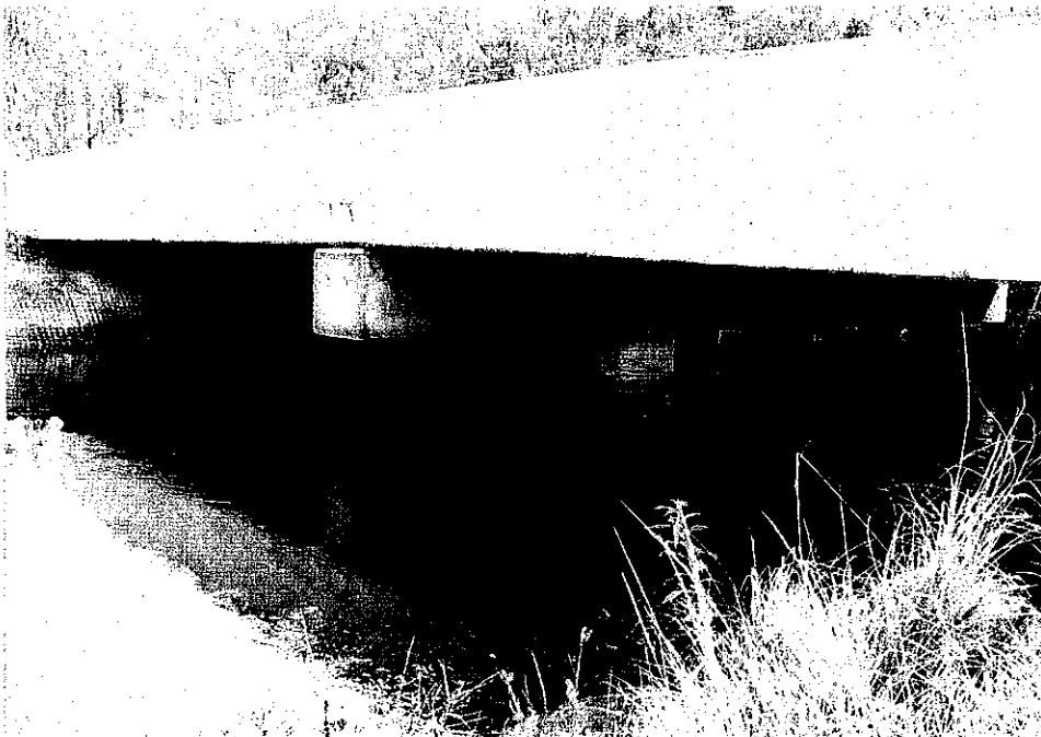
View southeast at Daughtrey Creek Bridge on Nalle Grade. Bridge is approximately 10 times larger in cross section than upstream culvert constriction.
