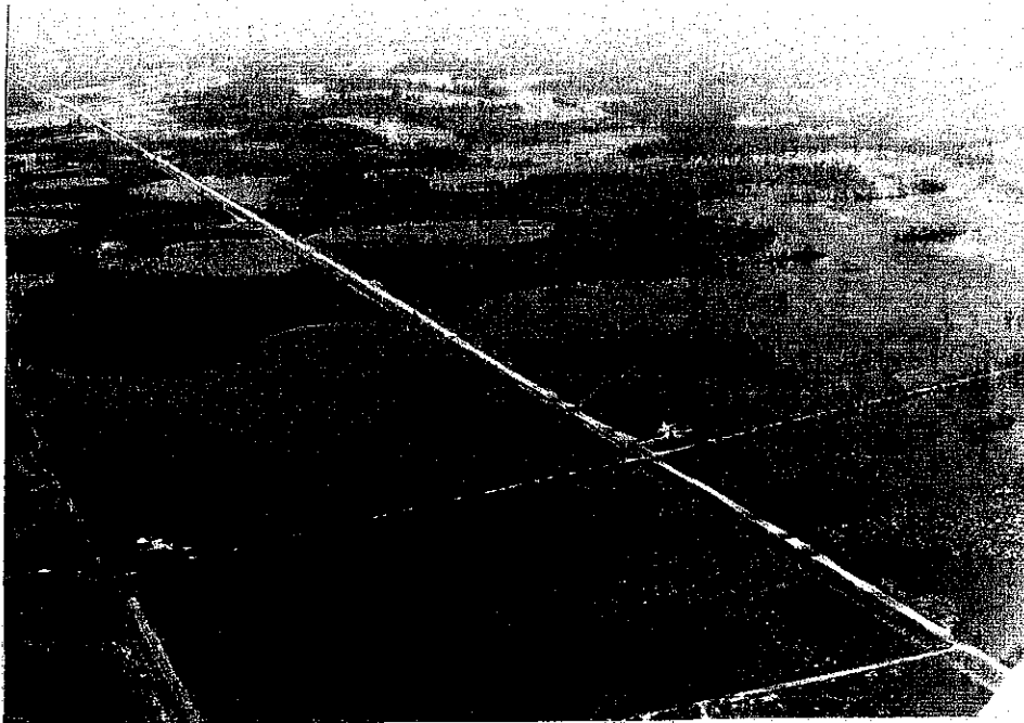
View northwest along Oil Well Grade near intersection of old Railroad Grade March 21, 1983. Typical flooding conditions. Note breaches in road at arrow.
