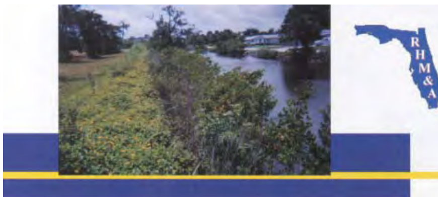
Figure 191: Stepped GeoWeb shoreline, Vero Beach Florida 1994.
